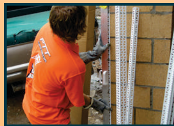
Suction will hold the trim in place & the levels will keep it straight
